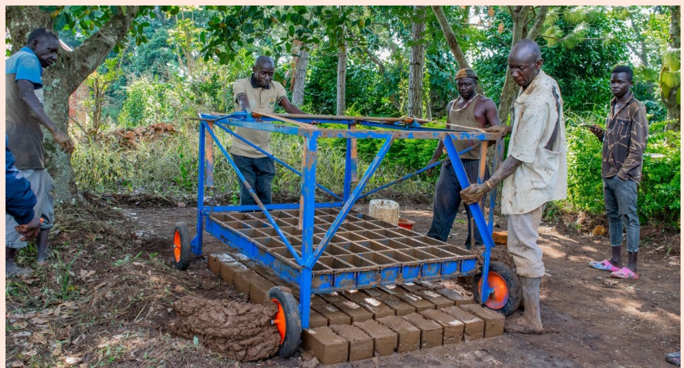
Beneficiaries of eco-brick machine from Kwonga Clan and MCODA producing quality bricks
